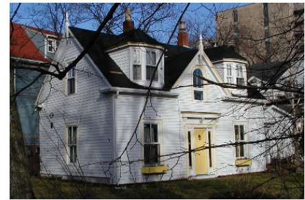
1029 Tower Road, Halifax, NS
